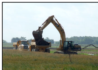
A backhoe loads excavated earth into a large off-road dump truck.
